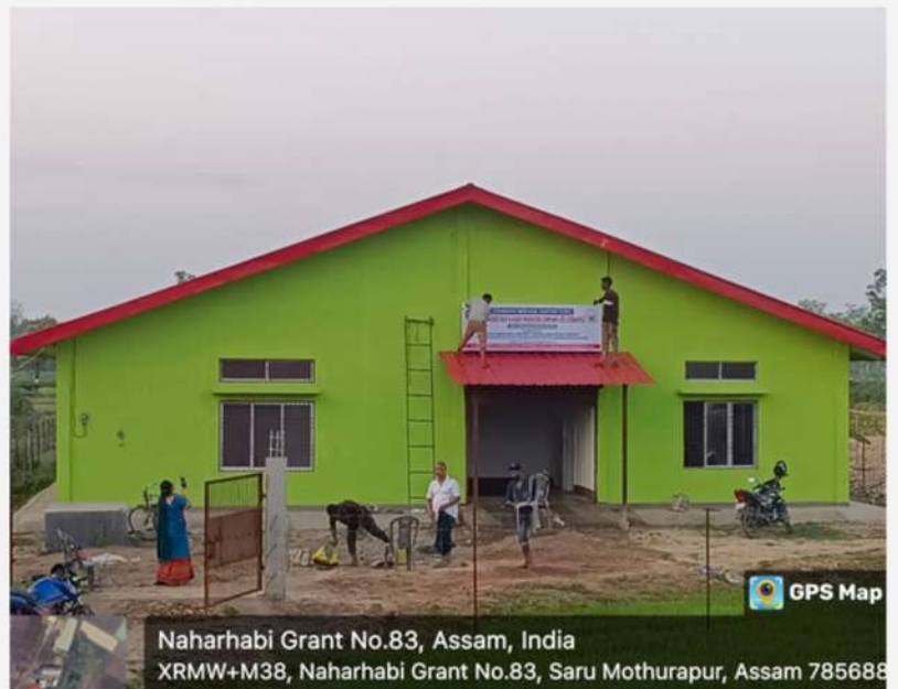
CSC constructed with support from APART
